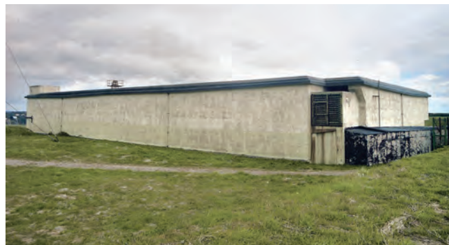
The R6 blockhouse at Hope Cove. Photo Nick Catford
